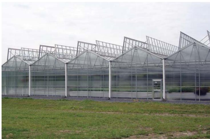
*Top: Natural, open-roof ventilation is an energy-efficient and practical system for greenhouse production. (Photo: Cravo Equipment) Bottom: Half-open roofs offer some of the same benefits as 100-percent open-roof greenhouses. (Photo: Nexus Corp.)*
