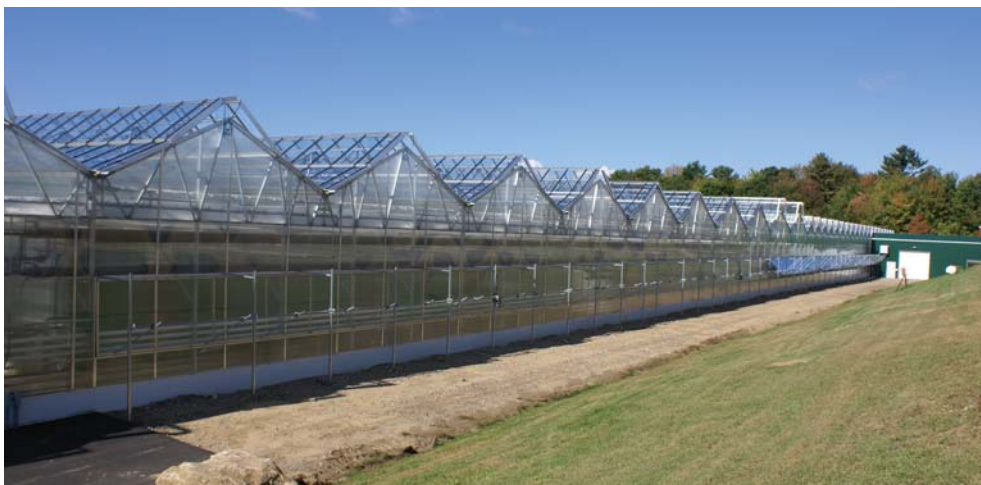
Dual-atrium greenhouses have half the gutters of open-roof structures and fewer working parts.
