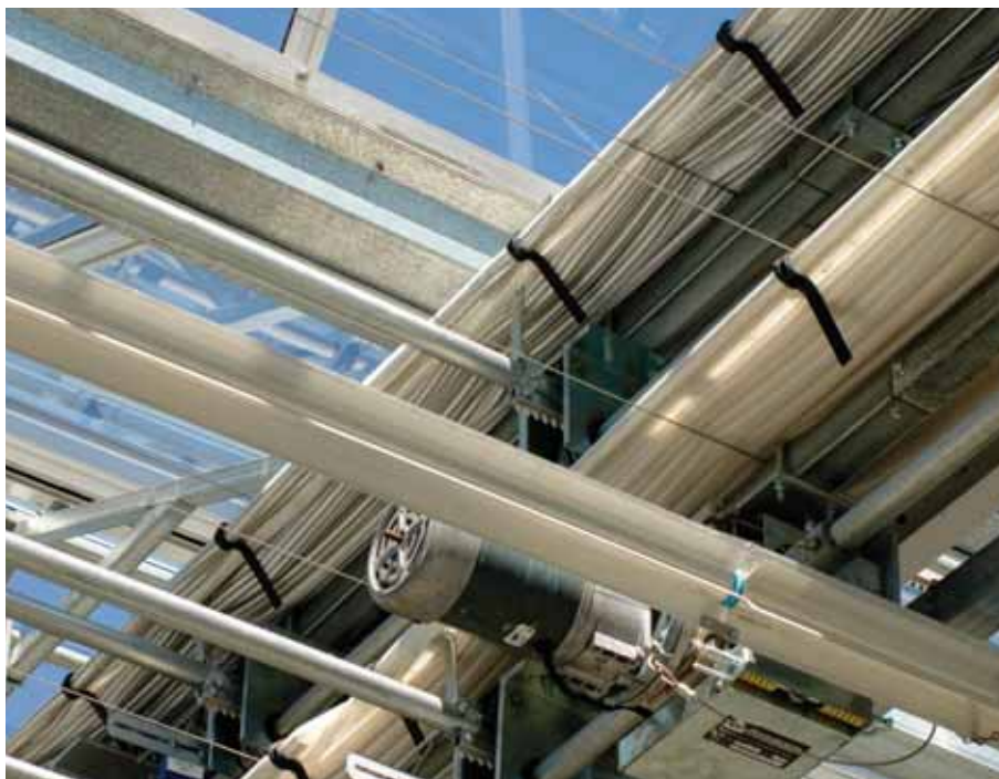
The Nexus Corp. dual-curtain system helps hold heat within the greenhouse.
